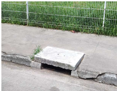
Q - Boca de lobo a demolir/selar
